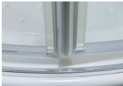
■ Threshold strip and bottom door seal
